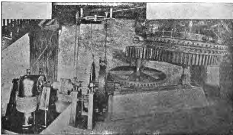
MACHINERY FOR OPERATING INCLINE.
