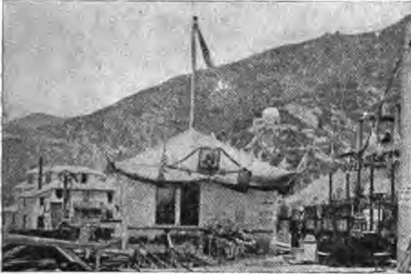
POWER HOUSE—CABLE INCLINE.
