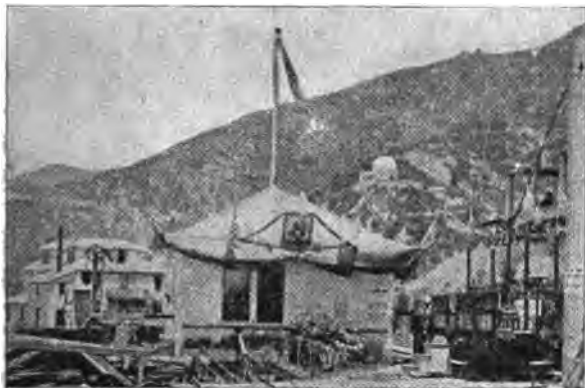
POWER HOUSE—CABLE INCLINE.
