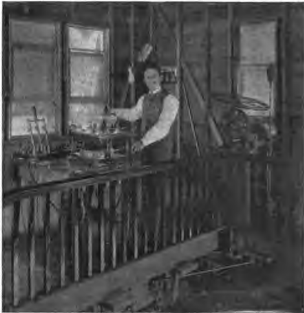
REGULATING APPARATUS FOR CABLE INCLINE, MT. LOWE RAILWAY.
