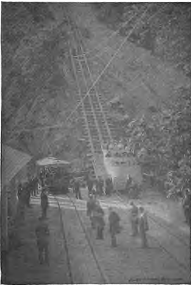
FOOT OF GREAT CABLE INCLINE OPERATED BY ELECTRIC MOTOR, MT. LOWE RAILWAY.
